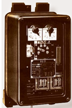
5 RG21, SIEMENS generator-differential-and stator ground fault protection
